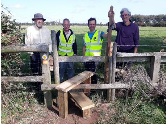
Waterstock stile rebuild
