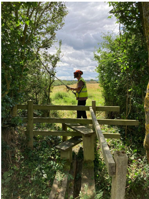
Putting the finishing touches to a footbridge and stile in Stanford in the Vale parish. We have reported the collapsing footbridge to OCC.
