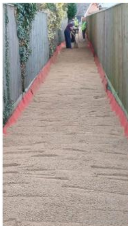
Gravel spreading and compacting
