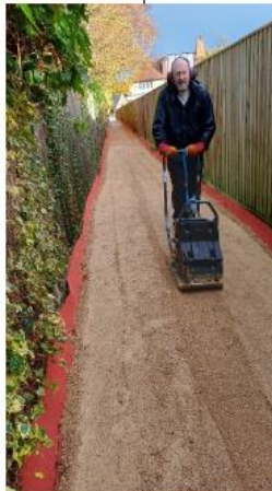
Gravel spreading and compacting
