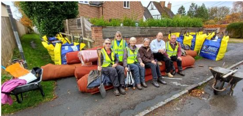
Preparing to start path work after carpet and gravel materials delivered
