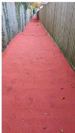
Carpet laying with overlap joints
