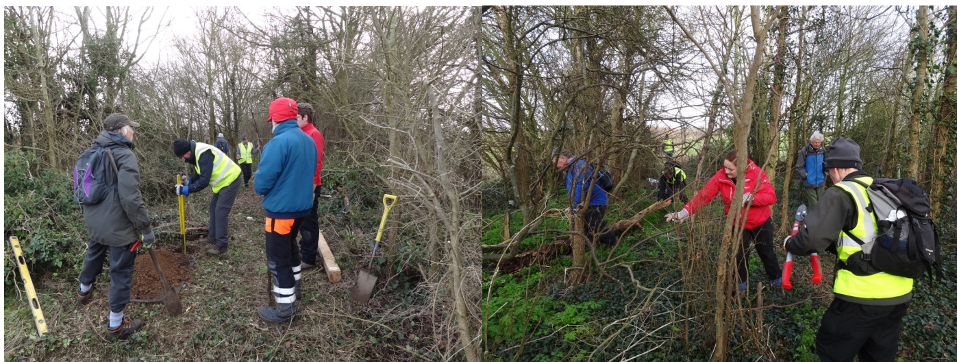
VPV working at Forest Hill to clear a path and install waymark posts. (Photos J Parke)
